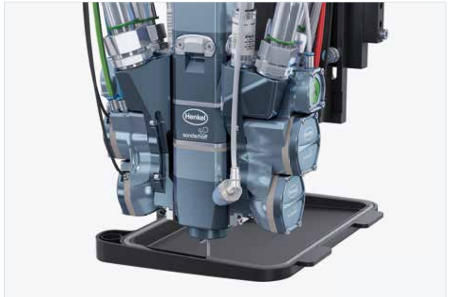
Dosing application of PU sealing foam into the cover groove of the battery housing via the CNC-controlled mixing head
