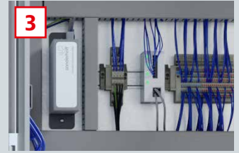
Modular "IPC control system" with Powerlink
