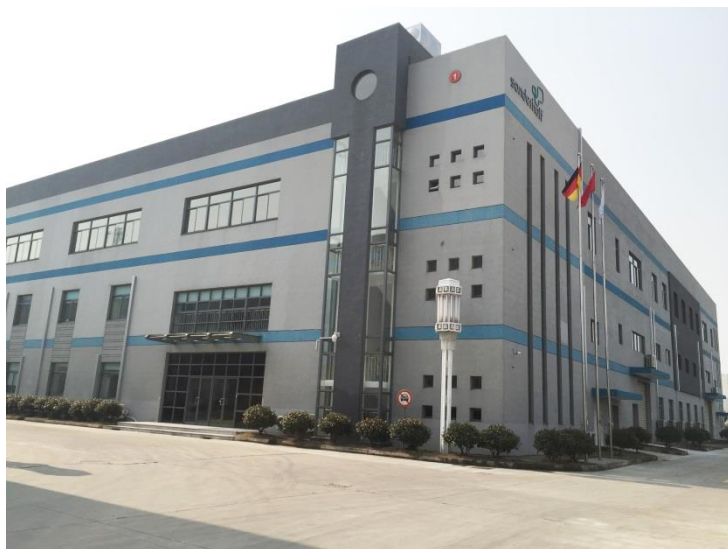
Location of Sonderhoff (Suzhou) Sealing Systems Co. Ltd. in the Suzhou Industrial Park, 215126 Suzhou. (Source: Sonderhoff)
