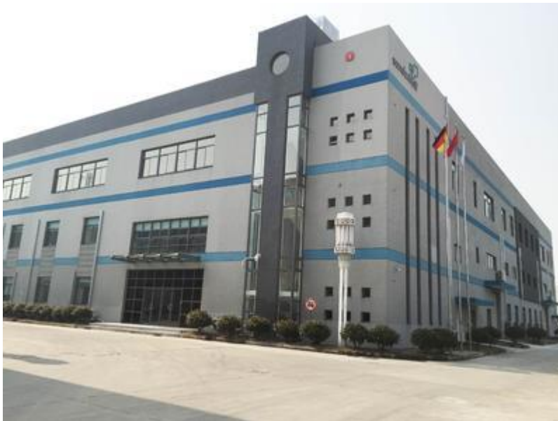
New location of Sonderhoff (Suzhou) Sealing Systems Co. Ltd. in the Suzhou Industrial Park, 215126 Suzhou
